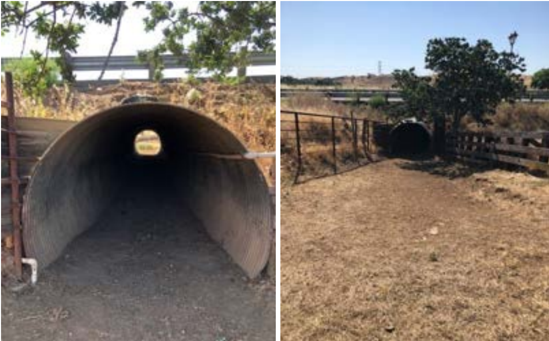
Photo: Existing Cattle Crossing under Marsh Creek Road near Camino Diablo Road
